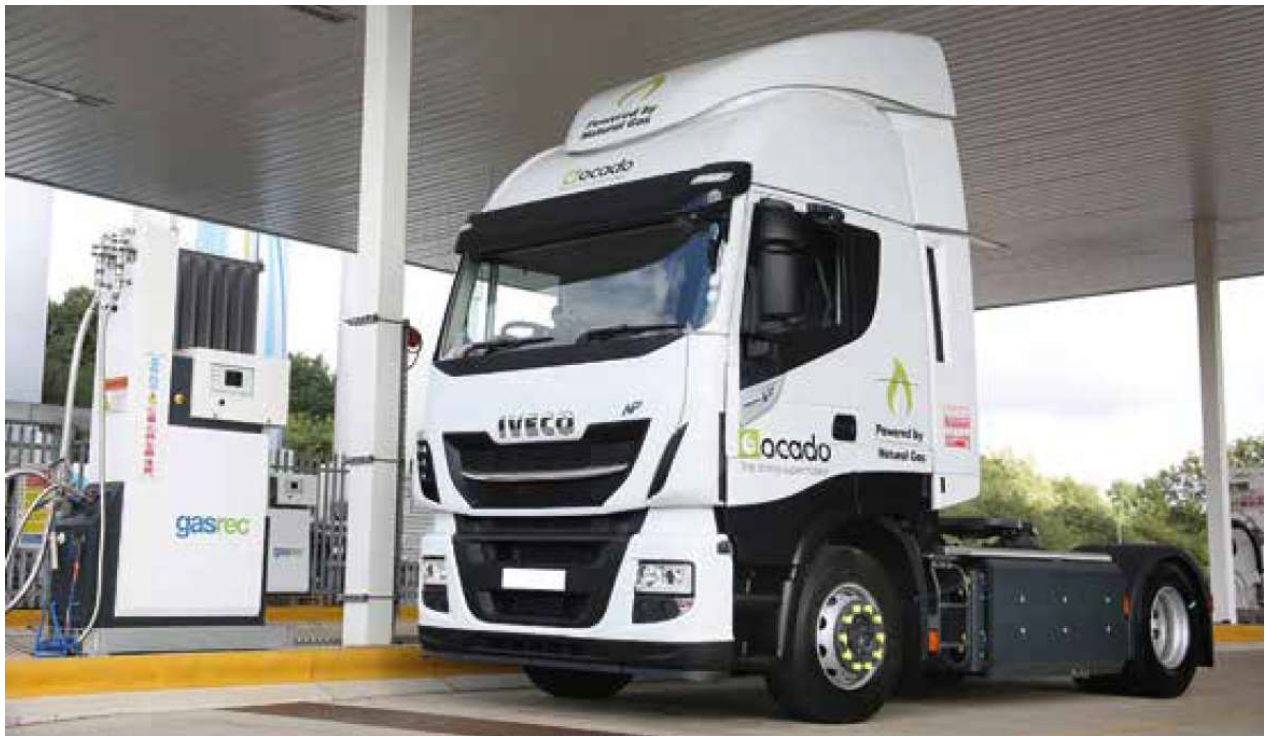
Figure 4-3 Ocado's Warwickshire UK CNG Refuelling Station, built by Gastec
