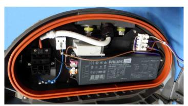
Photo 3. Luminaire geartray.
